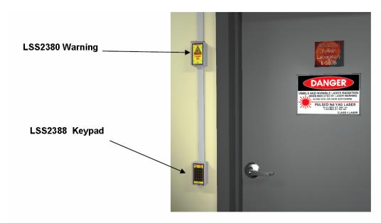
The front door is shown from the exterior. The LSS2380 Warning module is the starting point of our system. Authorized laser workers can bypass the door interlock by entering a pass code.
